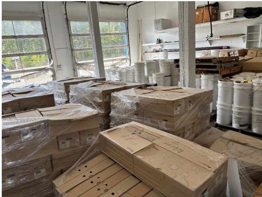
Figure 12-3 Blue River Pulp Storage Building
